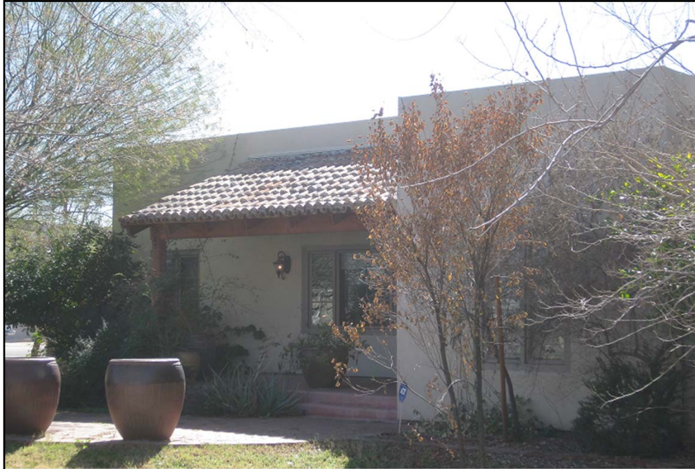
Burket House (1945) 501 West 5 th Street
